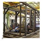
Structural steel is the most popular framing material for non-residential buildings in the world. Steel members, commonly referred to as beams and columns, form the skeleton of the building supporting all of the other components of the building.
