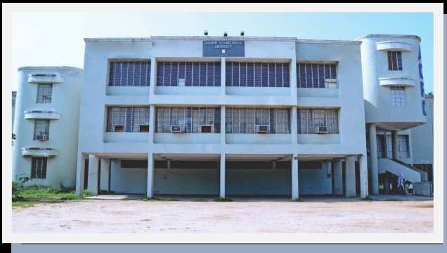
Admission Committee for Professional Courses Building, L.D College of Engineering Campus, Navarangpura, Ahmedabad -380 015 - Gujarat Phone: 079-2630 0499, 079-2630 0599
