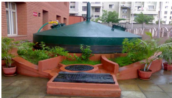
Bio digester of cow dung to produce bio gas as fuel
